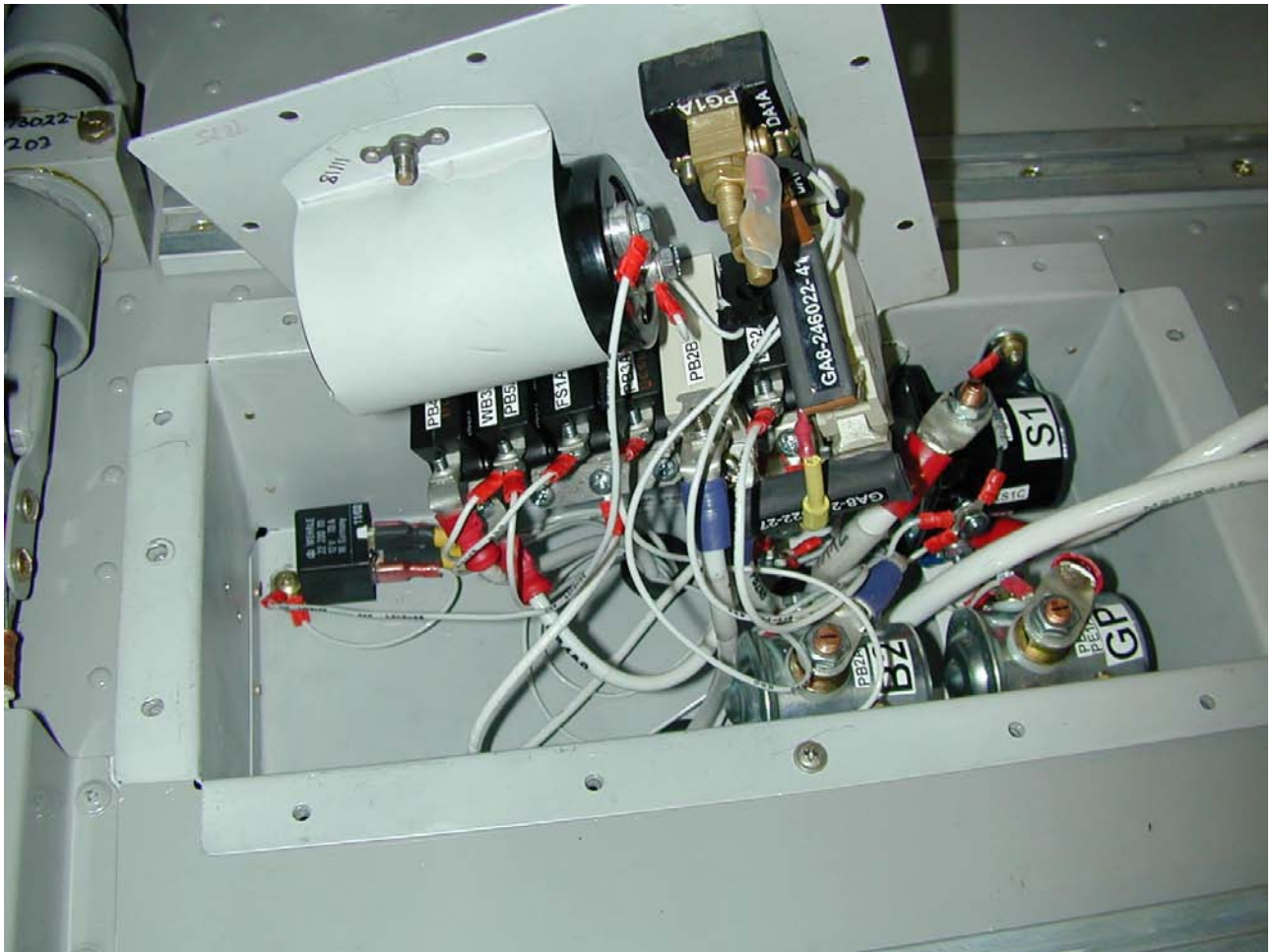
Figure 8-2 Capacitor, solenoid box installation
